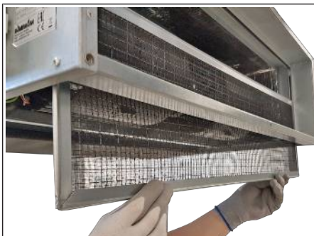
Afb. 55: Filter eruit trekken
